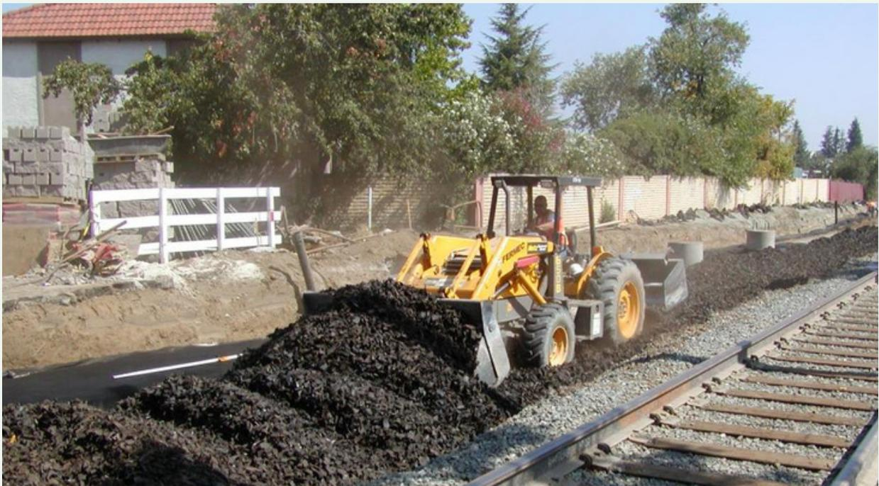
Tire-derived aggregate from recycled scrap tires can help reduce vibration and noise from trains.
